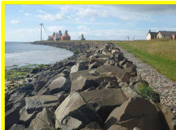
*Rock revetment with gabion baskets at rear (/4001C01)*
