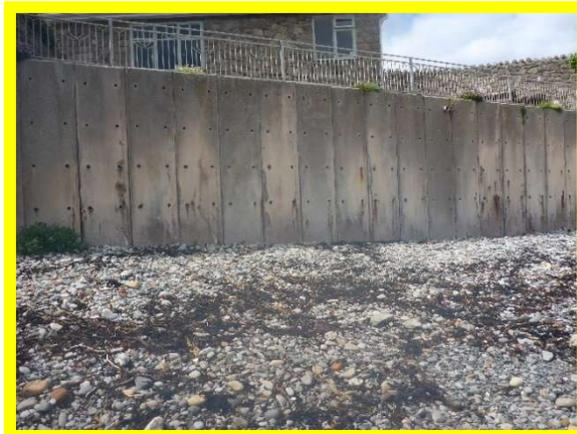
*Precast vertical seawall in good condition overall – minor cracking observed. (/1701/C31)*
