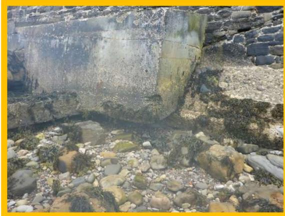
*Undermining of seawall at Beadnell North (Nacker's Hole) (/1701C36)*
