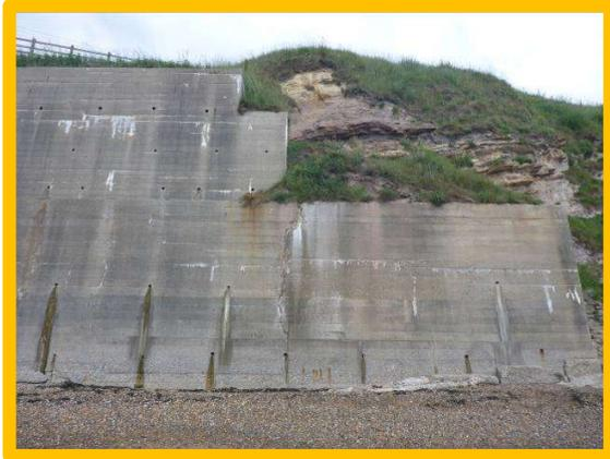
One of three notable vertical cracks in the sea wall (/4401C17)
