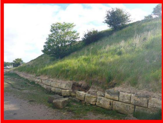
*Displaced blockwork in wall at Church Hill (/2801C13)*
