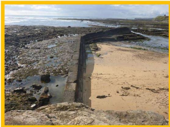
*Green's Haven Breakwater remains in poor condition but still retains beach sand (/0701C04)*
