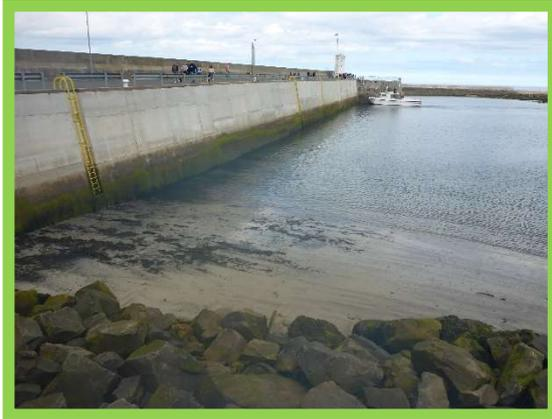
*Concrete encasement and cope repair to inner face of north breakwater. 1701/C09*
