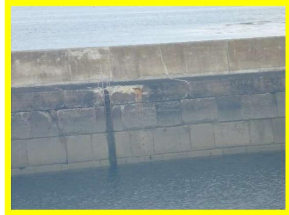
1701/C21 Some spalling visible on concrete cope.
