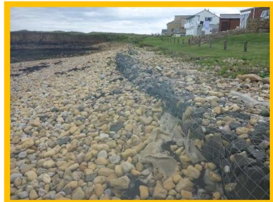
*Damage to gabion basket wall at (Lady's Hole) gabion wall – partially submerged to high sediment levels. (/1701C40)*
