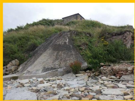
*1101/c04 2020 Outfall and concrete slope protection, cracked and minor undermining.*
