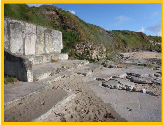
*Short seawall with active breaking-up apron (/0701C07)*
