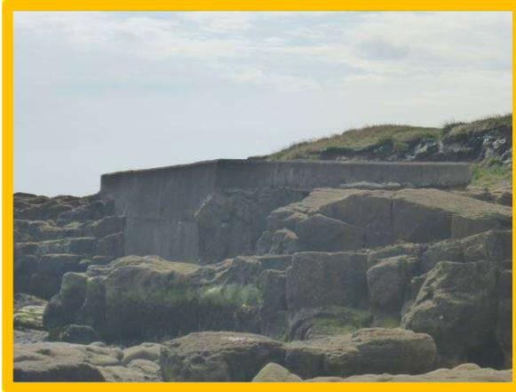
*Seawall with undermining and outflanking (/3501C08)*
