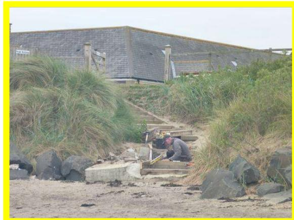
*Access steps being replaced through dunes at Low Hauxley (/3201C02)*
