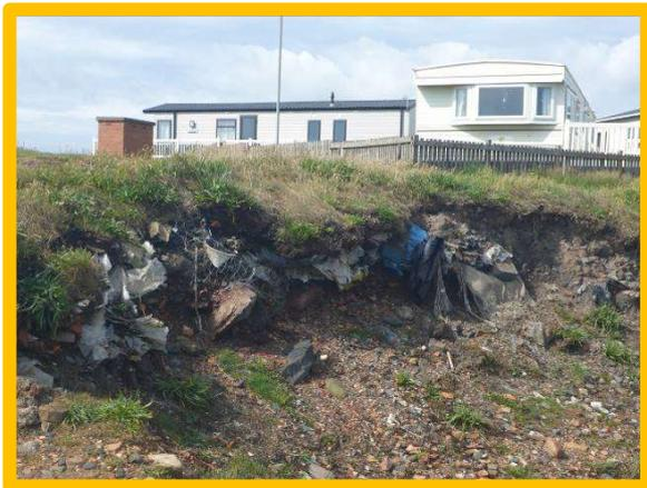
*Refuse buried in eroding coastal slope above seawall (/3501C08)*
