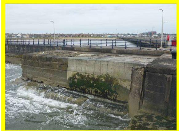
*Repairs at junction of South Pier and South Jetty (seaward face) made in 2018 (/3101C01)*
