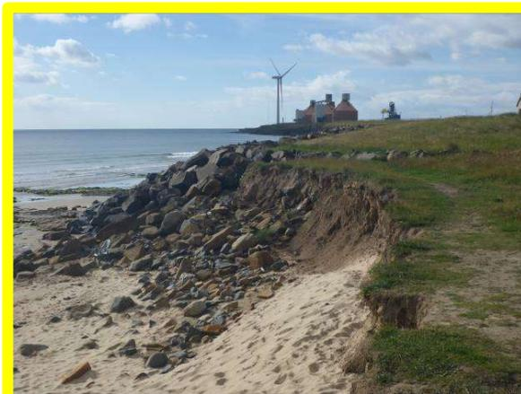
*View of terminal erosion at northern end of rock revetment (/4001C01)*
