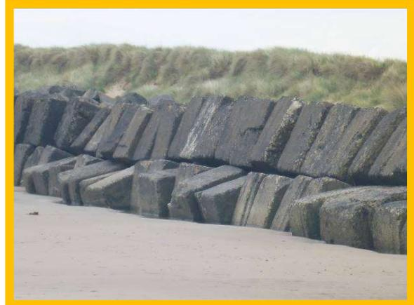
*Rotational displacement at southern end of concrete block revetment (/3201C04)*
