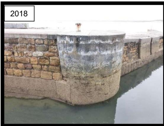
*Undermining of Beadnell Harbour wall (inner face of southern wall) 2018 (1701C51)*
