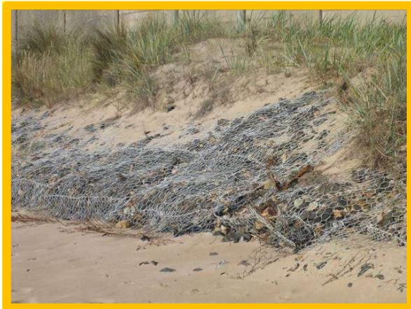
*Failing gabions protecting very narrow strip of dunes (/4201C03)*
