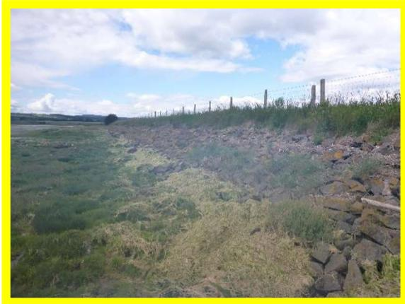
1401C22 – Section of evenly profiled, well graded revetment
