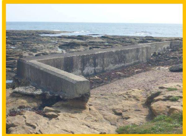
*Seawall with undermining and outflanking (/3501C08)*
