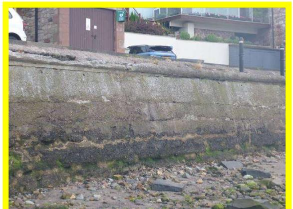
*Local failed section of river slope revetment/wall Local damage to wall coping (/0801C07)
