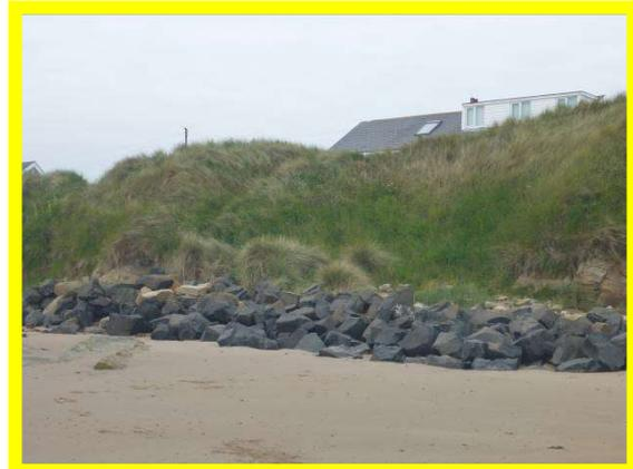
*Loosely placed rock armour at Low Hauxley (/3101C14)*
