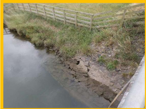
*1401/C01 – 2020 undermining of edge protection.*
