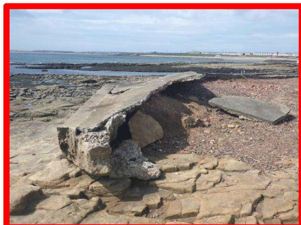
*Second length of seawall with undermining and outflanking (/3501C10)*
