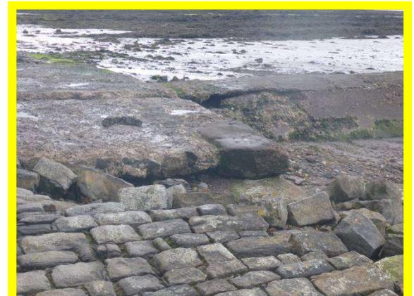
*Local failed section of slipway over foreshore Local failed section of slipway over foreshore
