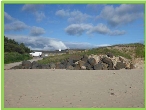
*Reinstated and improved rock revetment protecting slipway (/3901C05)*
