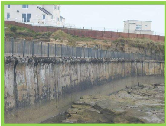
*Seawall in good condition despite rust-staining (/3101C05)*
