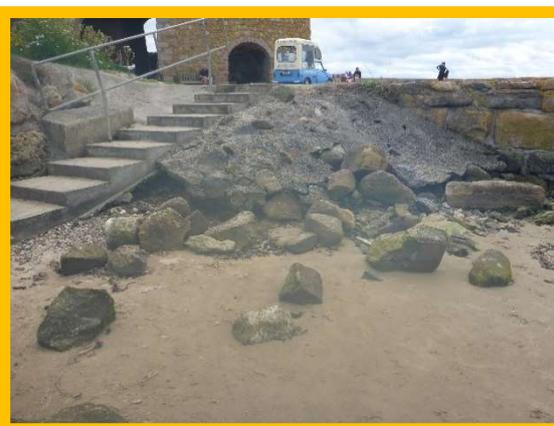
*Undermining and partial collapse of grouted stone revetment adjacent access steps. (1701C53)*
