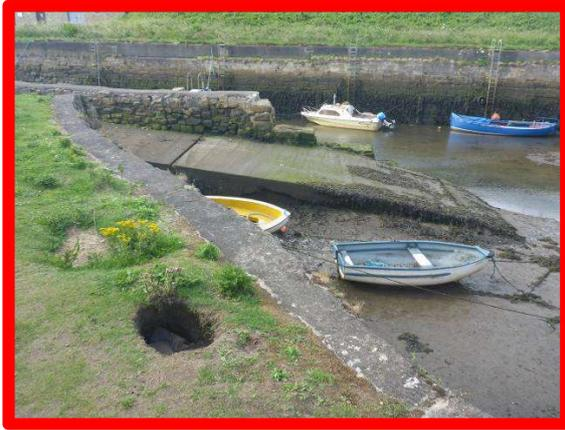
*Undermining at toe on inner face of boat ramp (/4401C05) – locally very poor*
