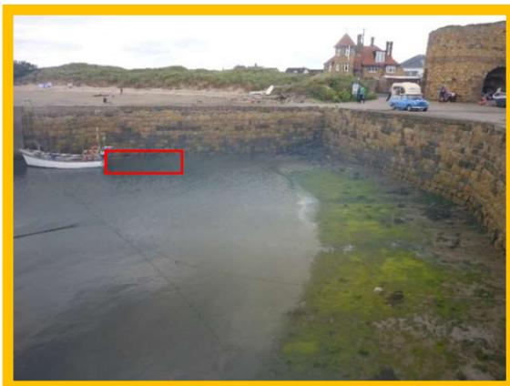
*Missing blocks at Beadnell Harbour wall (inner face of northern wall) (1701C52)*
