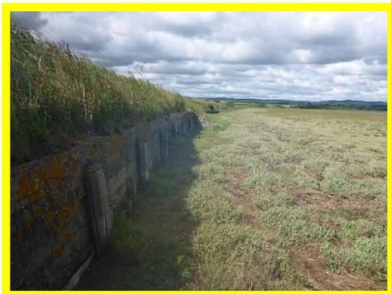
*1401C98 – retaining structure in fair condition. Rotten timber support posts and minor rotational movement.*
