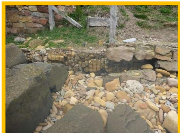
*Damage to retaining wall adjacent lime kiln. Possible slumping of slope to rear (/1701C45)*
