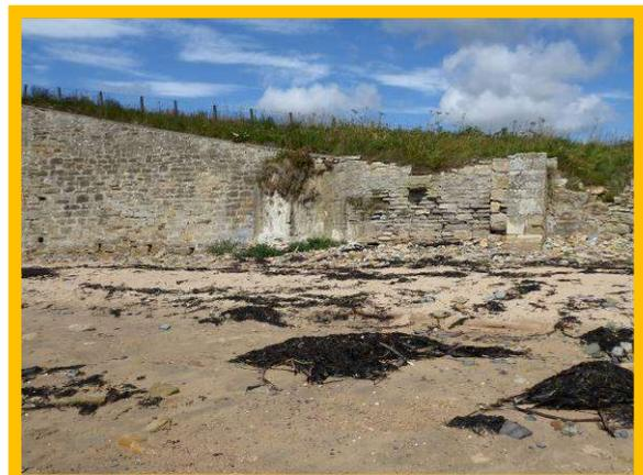
2501/C01 masonry wall in poor condition.
