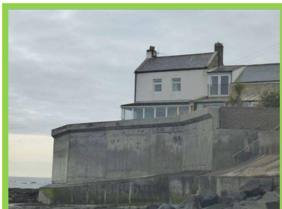
*Substantial seawall in overall good condition (/3101C07)*
