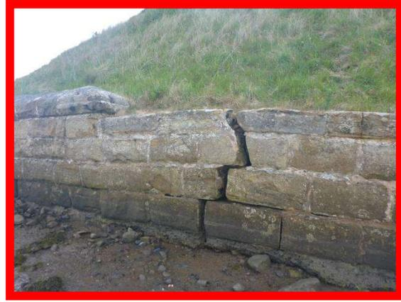
*Cracked section of wall at Church Hill (/2801C13)*
