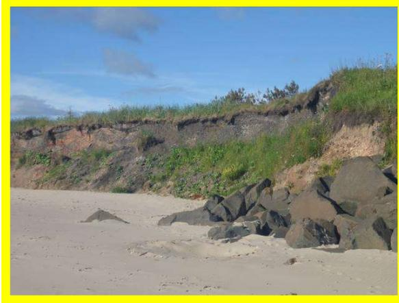
*Erosion of cliffs at terminal end of rock revetment (/3901C03)*
