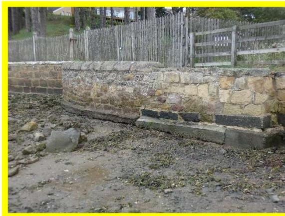
*2801/C10 Local undercutting of concrete toe to repaired section*
