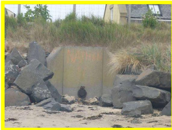
*Outfall with large headwall at Low Hauxley (/3201C02)*
