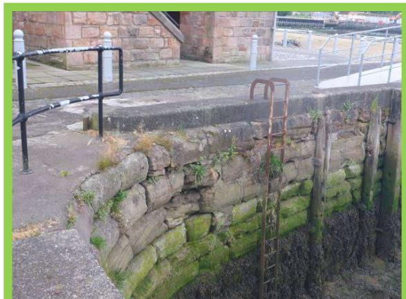
*Masonry quay walls in dock area in fair overall condition with some open joints, cracks and abrasion (/0801C03)*
