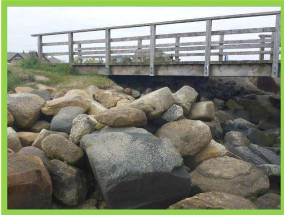
*Rock and boulders provide additional erosion protection at root of linkspan bridge (/3001C07)*
